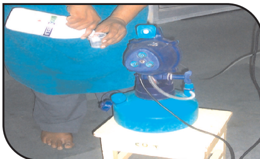
Fogger Machine in use
